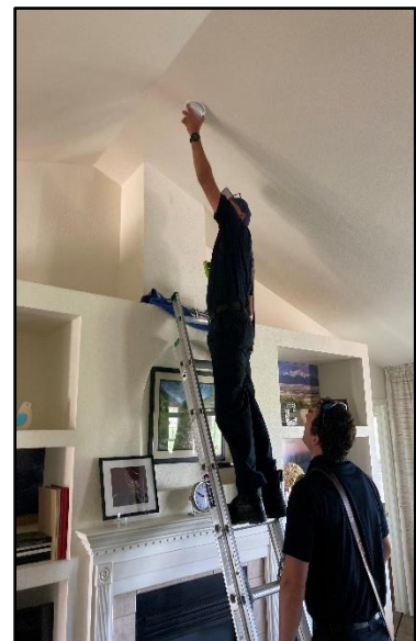
Crews checking a smoke detector.
